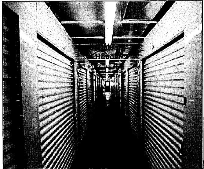
q. An interior corridor with flush headers has a fixed height with a gap between the corridor and purlin. The gap varies depending on the location of the corridor. • The lights should be centered in the hallway. • Material used to support the lights are by others.
