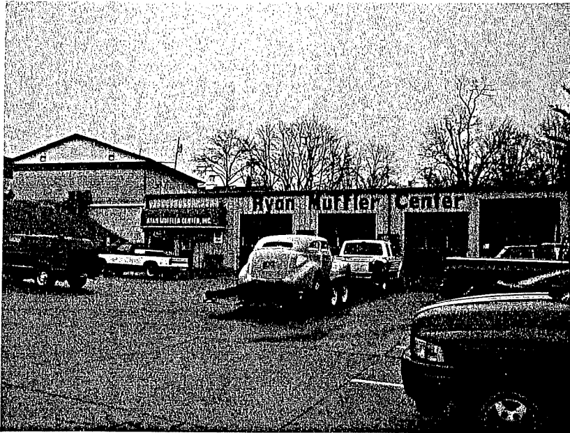
EXISTING BUILDING FRONT
