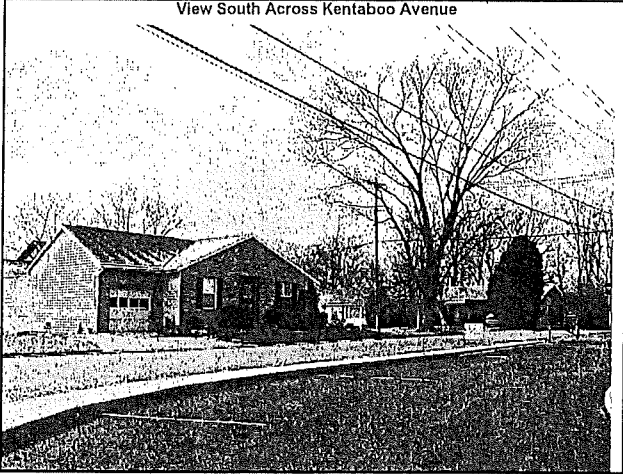
View South Across Kentaboo Avenue
