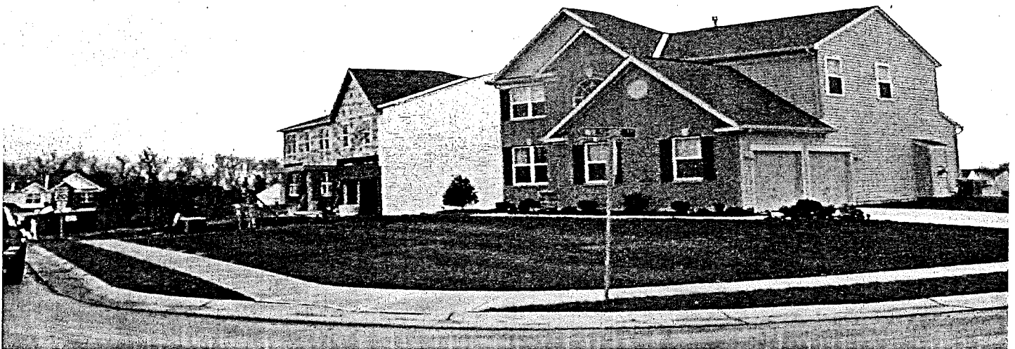
View of Site from Cherbourg Drive & Wilshire Court
