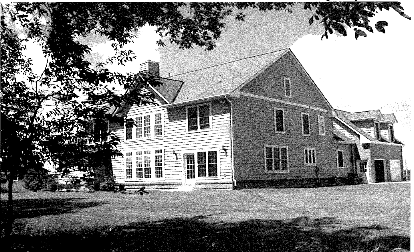
View of Adjoining Residence to the North
