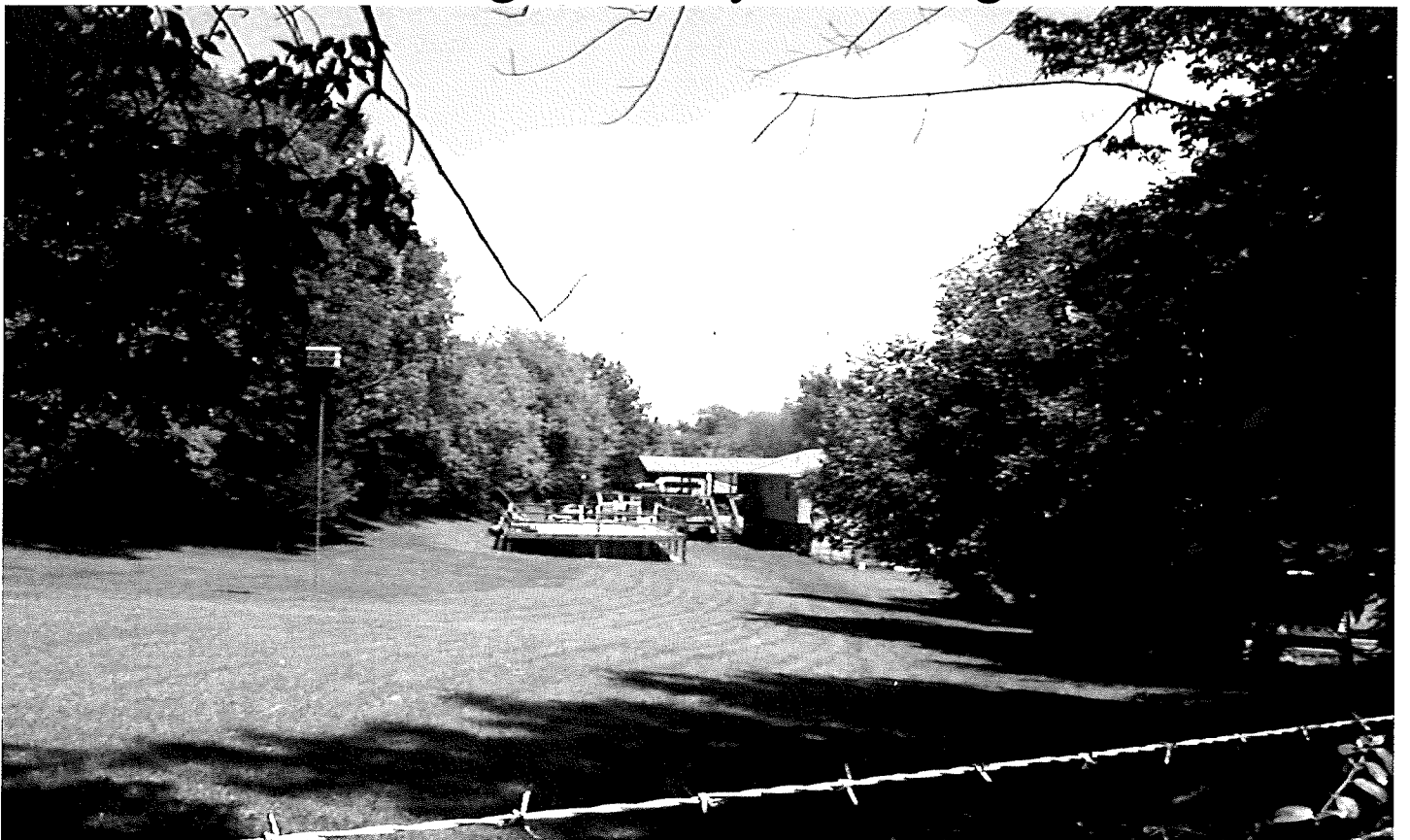
View of Single-Family Dwelling to East
