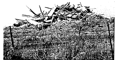
View from Tagher Residence driveway. 8 foot buffer mound and trees not present. Downed buildings in view for several months.
