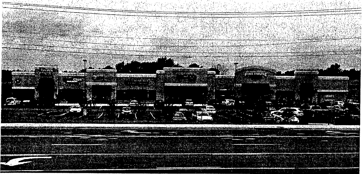
Houston Road Shoppes- Overall View (Drake*s unfinished)
