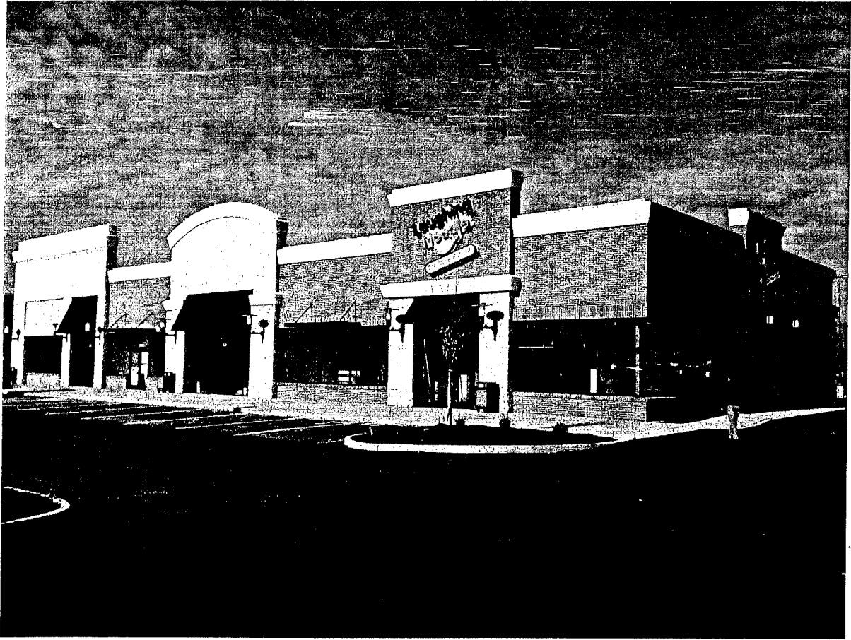
Houston Plaza- Overall View (tenant fit-ups still underway)
