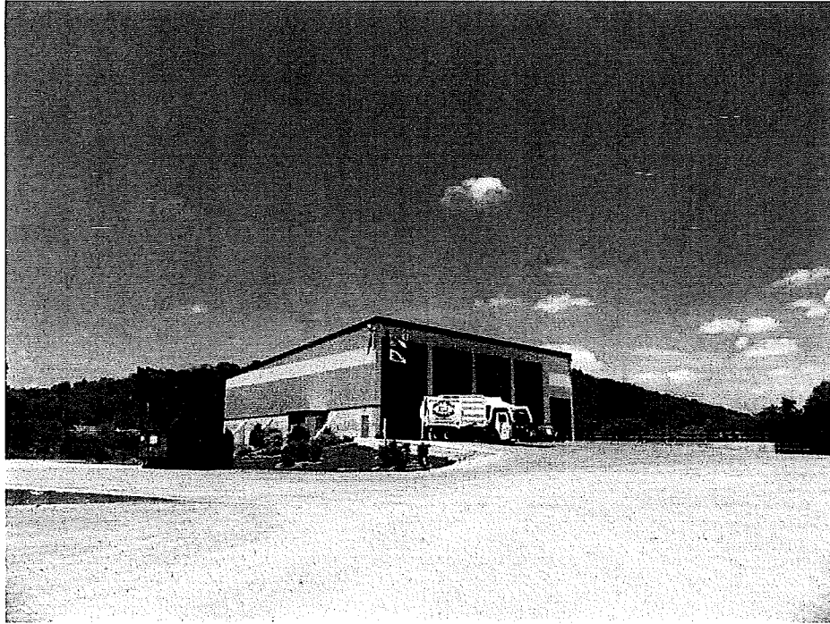
Side photo of an existing Bestway Transfer Station in Dearborn County, Indiana
