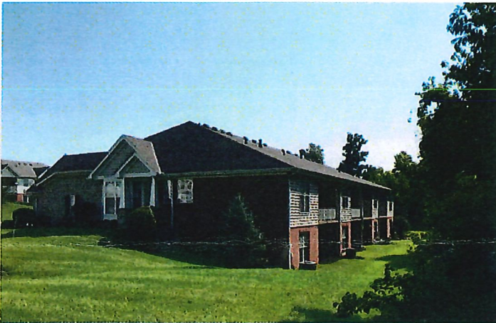
Side/Rear – Vinyl siding with more high profile areas enhanced with brick/stone wrap
