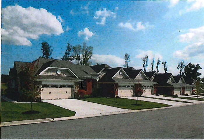
Front – Predominately Brick/Stone with some vinyl siding mixed in.
