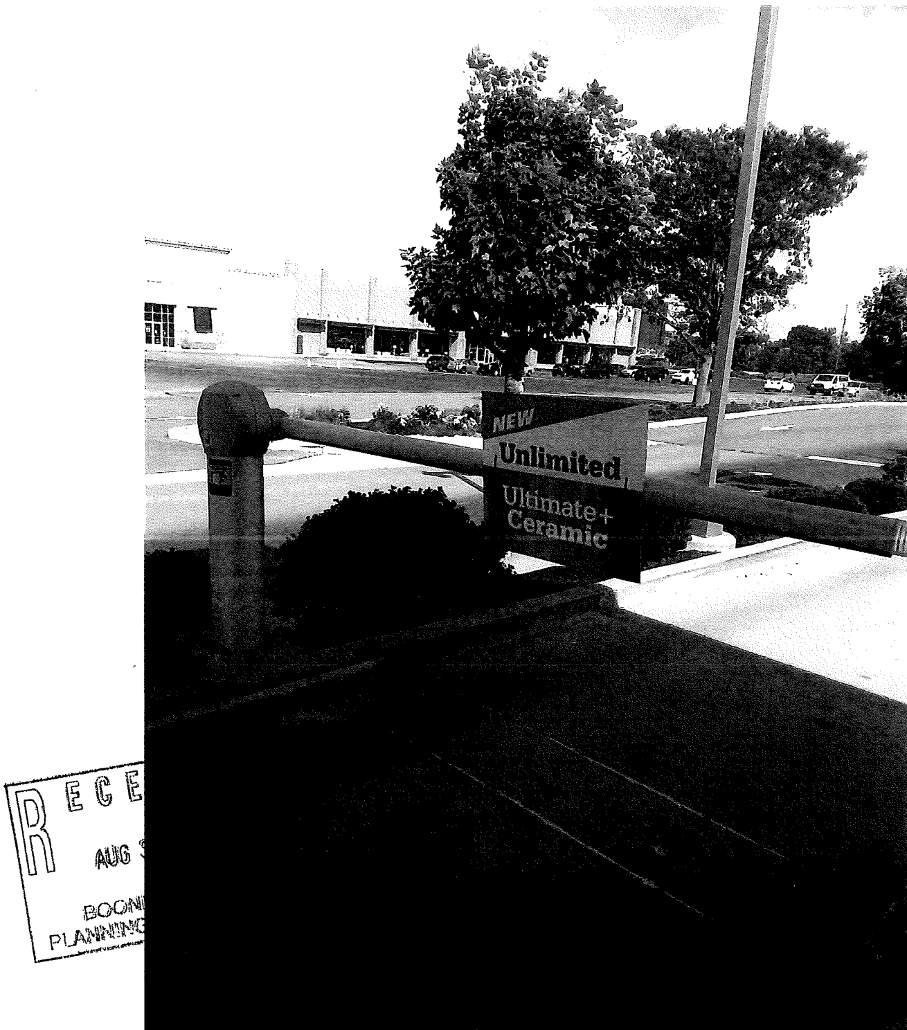
This picture is representative of the style of gate (barrier arm) that is being proposed for the Villages of Fowler Creek. The gate will be equipped with some form of a keypad or other system to allow residence to exit the site. The final selection of a gate and keypad is still being discussed with suppliers.
