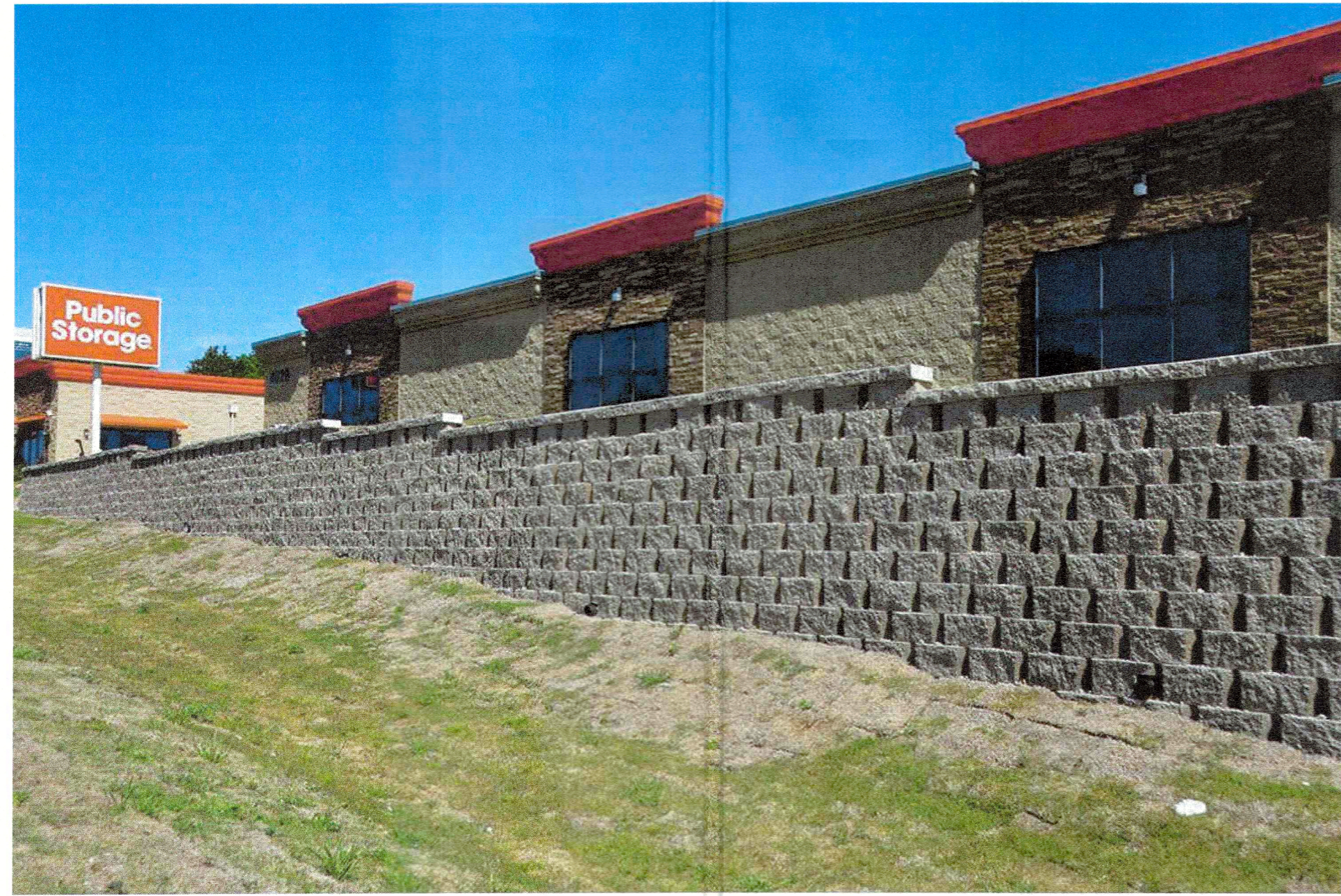
EXAMPLE RETAINING WALL
