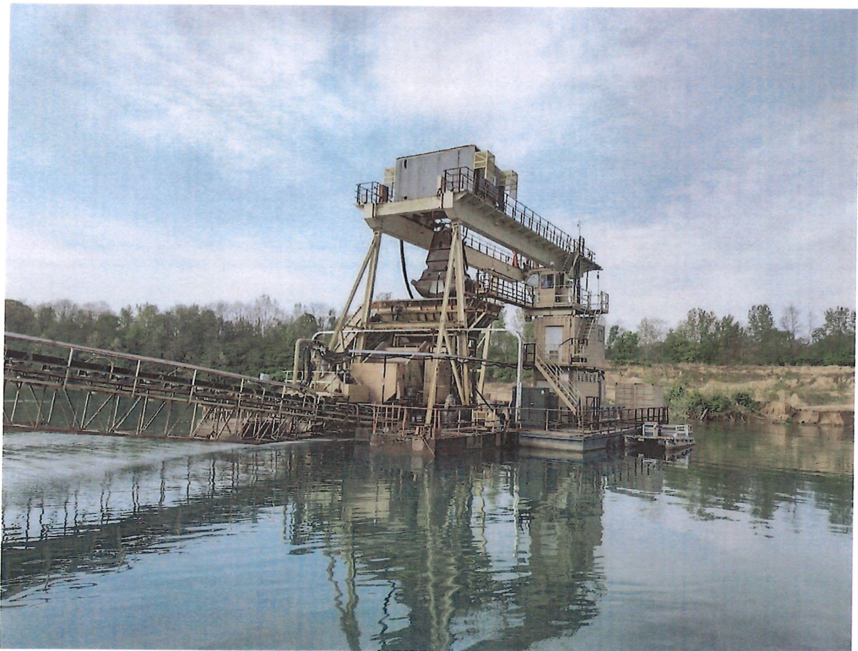
Figure 3. Rorh Electric Clamshell Dredge And Conveyor
