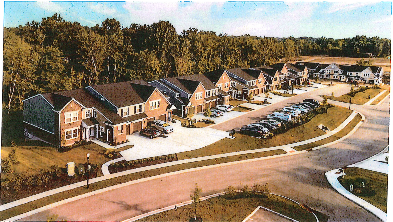
Existing Community Elevation
